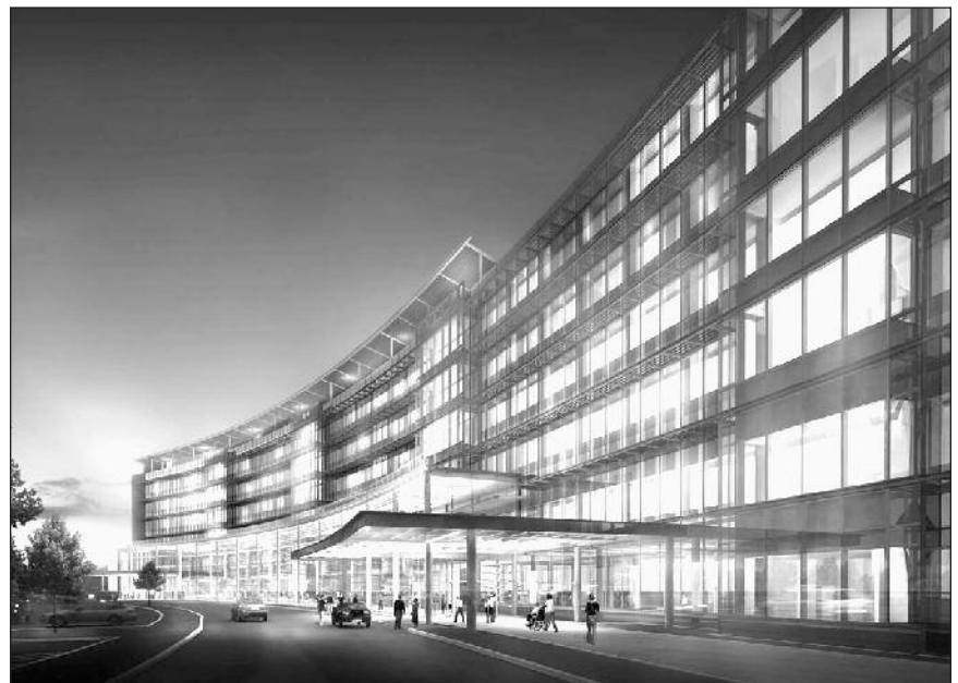
The new 636,000 square foot University Medical Center of Princeton at Plainsboro will contain 243 beds and state of the art diagnostic and treatment facilities. The medical center is scheduled to open in the summer of 2011.
