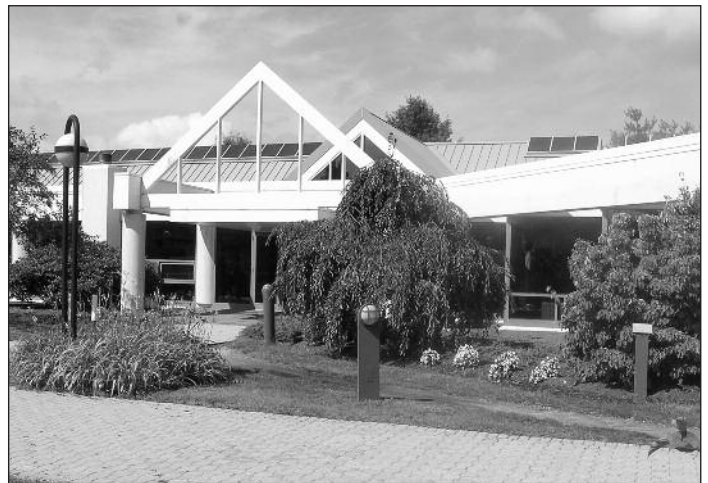
The existing 17,500 square foot Plainsboro Library will be renovated to serve as a recreation facility. Construction will start in 2010.
