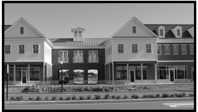
Construction of the Village Center continues to progress. The buildings shown above, which front on Schalks Crossing Road, will soon be occupied.
