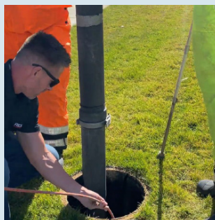
Vacuum removal of debris
