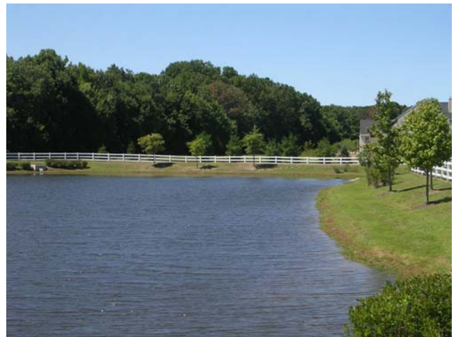
Stormwater Detention Pond
